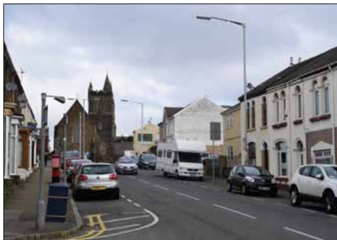
Figure 20: View north on Martin Street towards St John's
