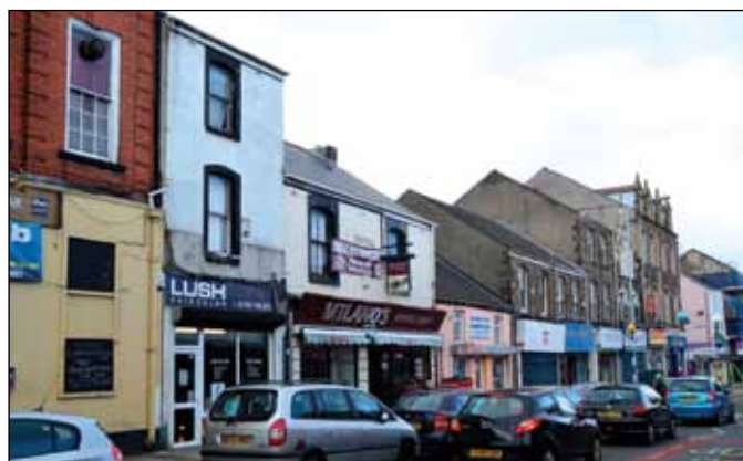
Figure 19: View north along Woodfield Street
