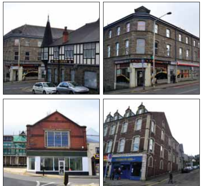
Figure 30: Examples of strong corner buildings
